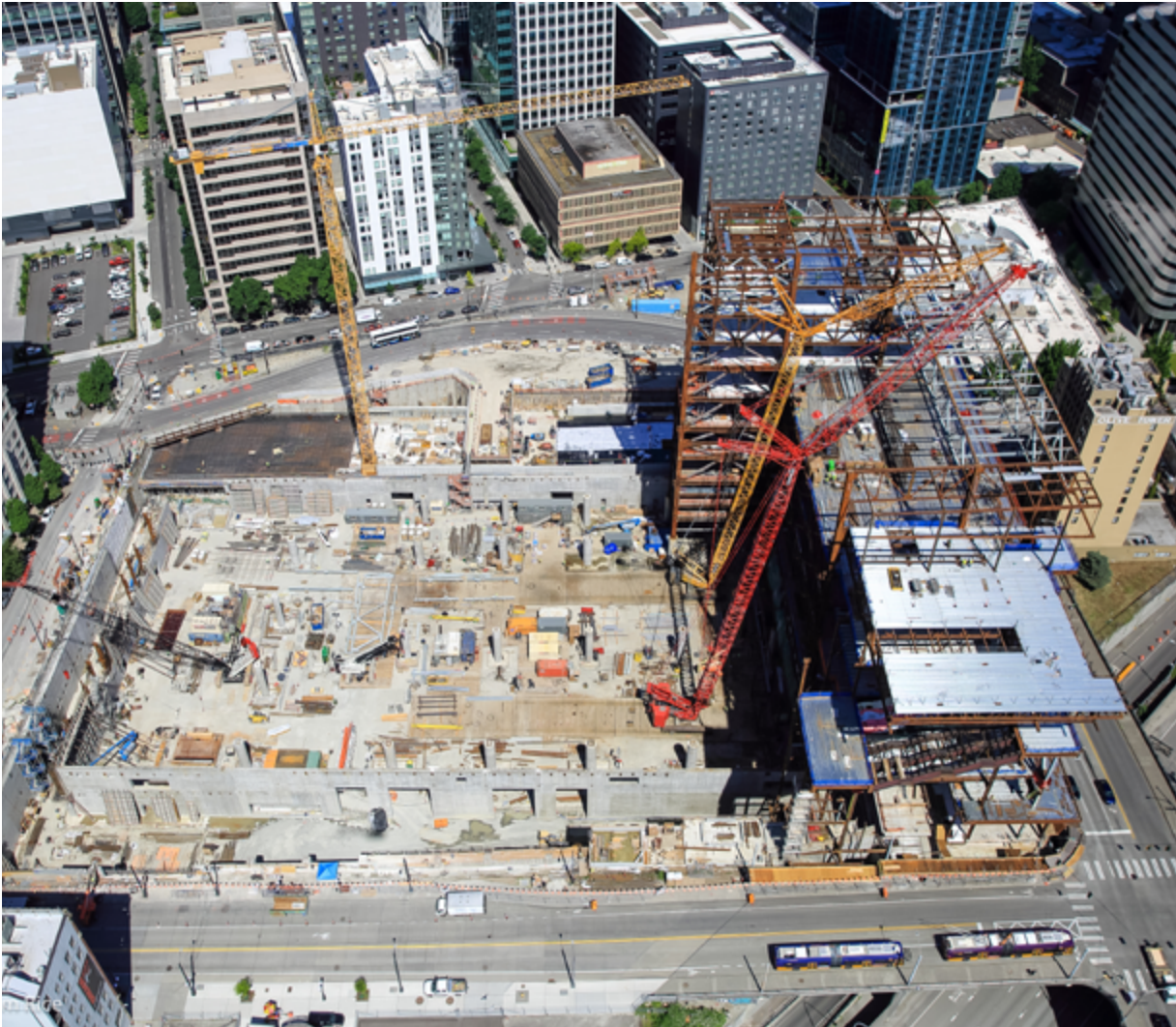
Summit construction photo illustrates the “billboarding” method.
